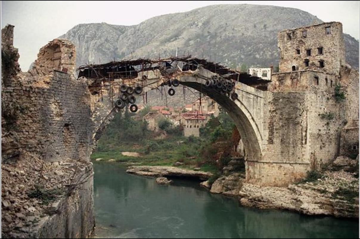
Picture 5: Old Bridge in 1993 before destruction
