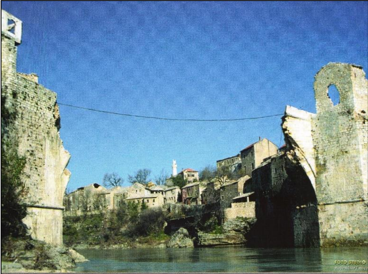
Picture 6: Old Bridge in 1993 after destruction
