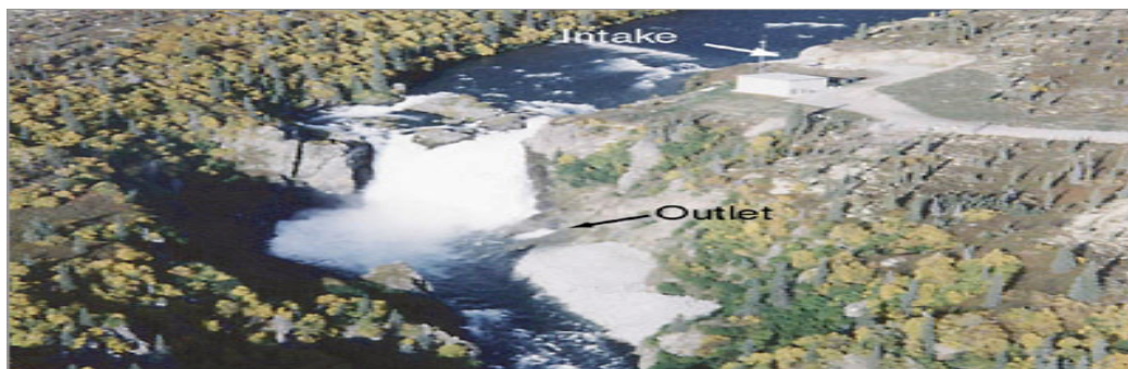
Figures 3: Diversion Dam. A form of diversion hydroelectricity plant in Alaska
