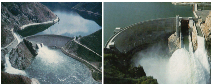
Figures 5: Gravity dam (to the left) and arch dam (to the right)
