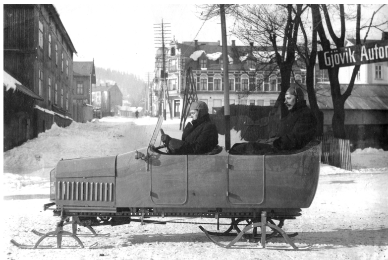
The automobile pictured in the centre of Gjøvik. The driving wheel at the rear of the automobile is clearly visible. (Picture from my own collection).
